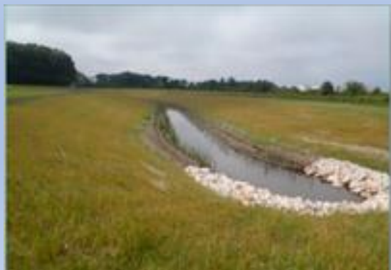
Skokie River daylighting – open channel with native plants
