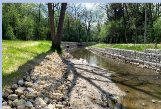
Skokie River streambank stabilization Lake Forest
