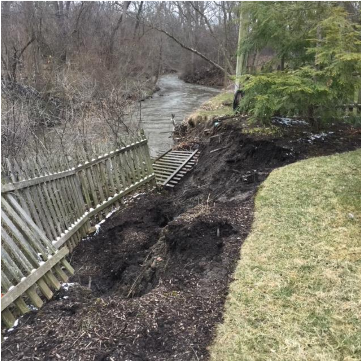
Lake Forest Emergency Repair April 2018
