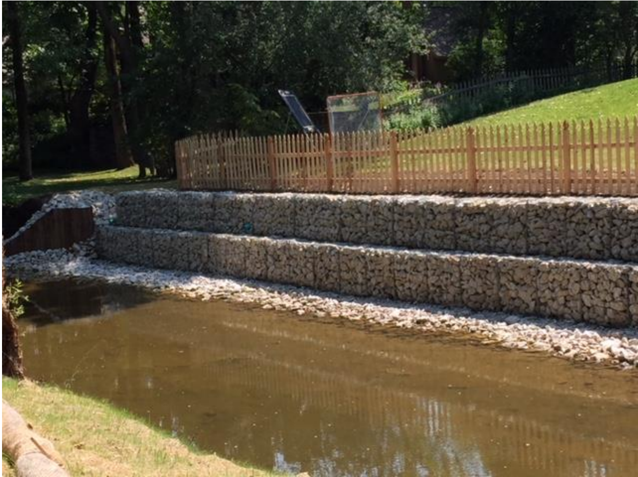
Lake Forest Emergency Repair August 2018
