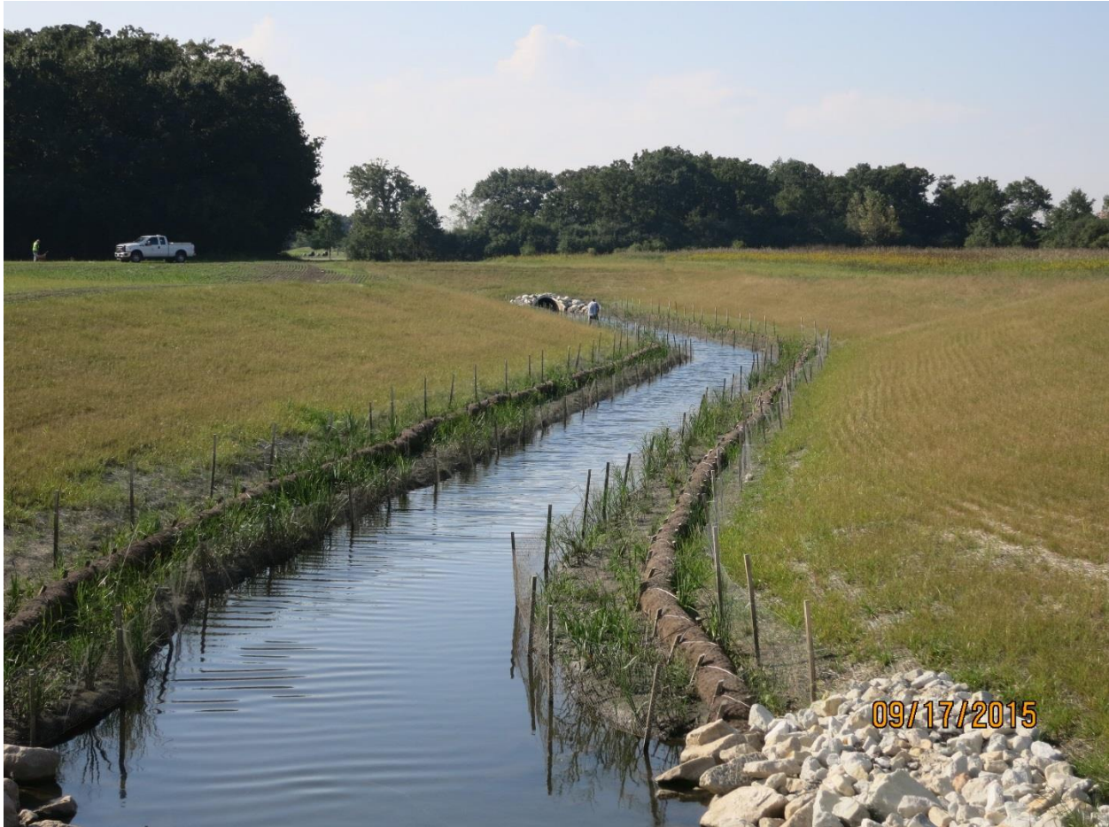
Proctor & Gamble 2-Stage Channel Project- North Chicago, IL; completed Fall 2015
